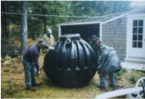
Crew carrying tank into place
