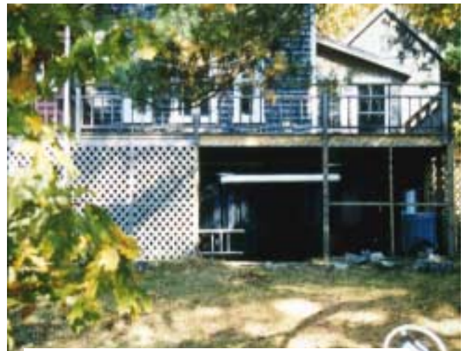
Tanks above ground but hidden from view under deck
